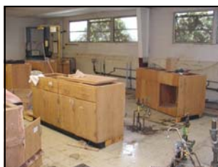
Demolition of the Enology Lab began in the Fall of 2005
