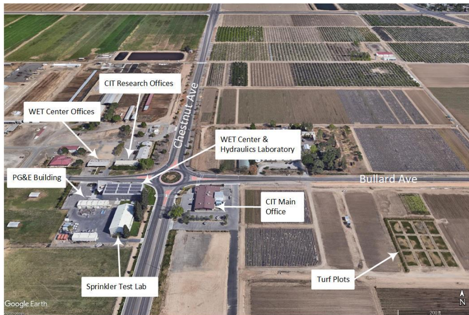
Figure 2 An aerial view of the of the CIT & WET physical facilities
