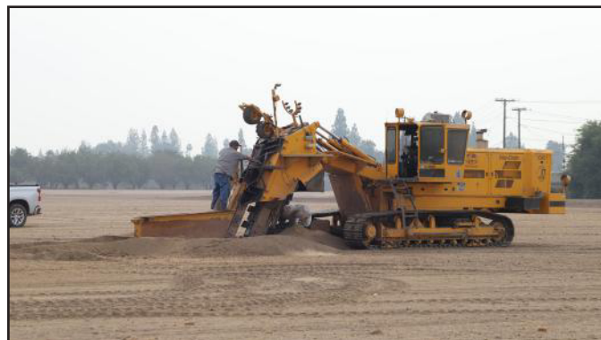
Lidco installed the perforated pipes with 12 feet deep using large trenchers
