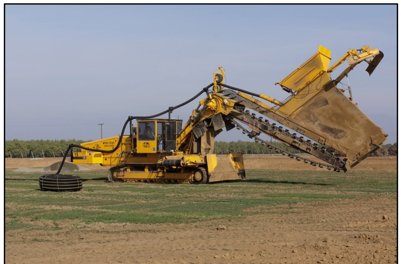
Trencher getting ready to install perforated pipe.
