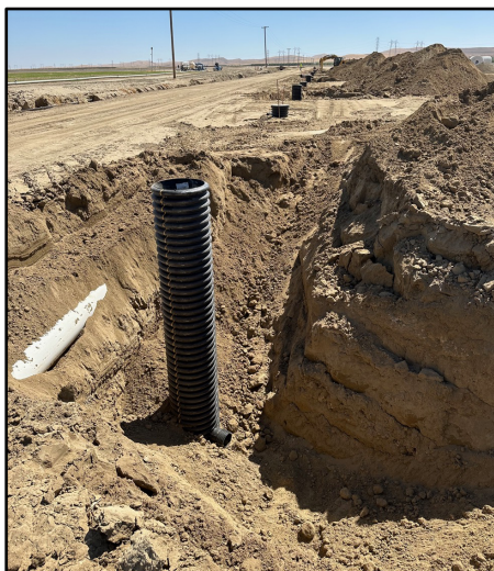
Standpipe Installation
