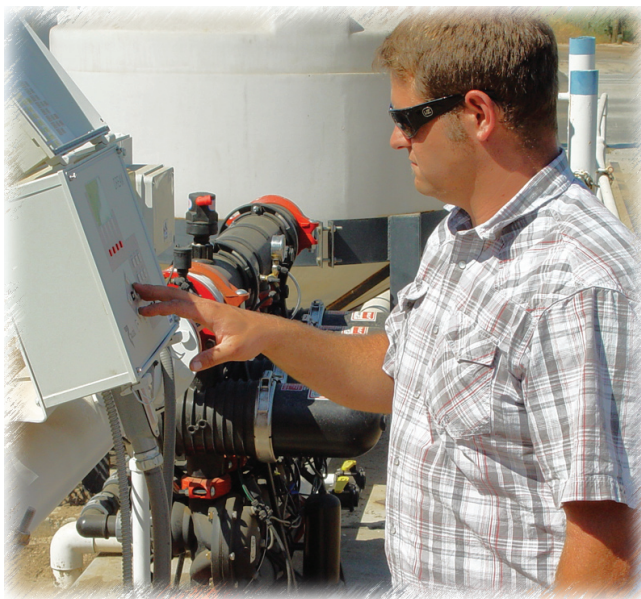
Fresno State plant science student Matthew Smith operates the main electronic controller for the Paramount Citrus Lab acreage on the university farm. The controller operates 10 valves serving 20 acres of several citrus varieties.
