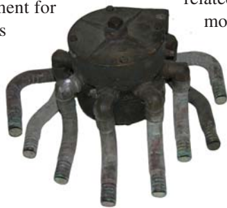
Spider valve? A residential main sprinkler valve dating from around 1925. Cast iron center supports copper tubes for attachment to sprinkler lines. Weight: Approx. 35 pounds. Manufacturer: Unknown.
