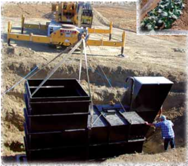
Left: 14-ton steel-framed weighing lysimeter and control room is installed in experimental field near Five Points, California.
