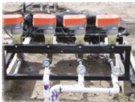
Custom-made manifold injects CO 2 gas into drip lines for application on strawberry plants.
