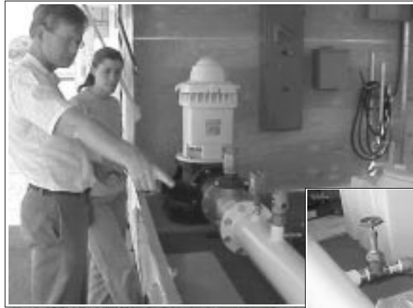
CIT education specialist Tim Jacobsen explains the functions of the new wellhead training trailer with backflow preventer to Joy Dias, field representative for the California Department of Pesticide Regulation. Photo below shows setup for a venturi injector unit.
