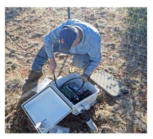
Figure 4.—Harry Hosler (from the Flagstaff office) carefully measures excess sensor cables to cut and stow in the climate station datalogger box.
